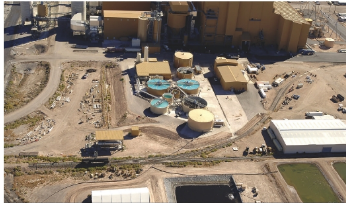
The Springerville Generating Station owned by Salt River Project, located in Springerville, Ariz. One of Arizona’s largest power entities, the coal-fired plant’s capacity as of December 2009 is 1560 MW. Photo: SRP.
