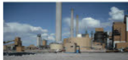
Springerville Generating Plant in northern Arizona
