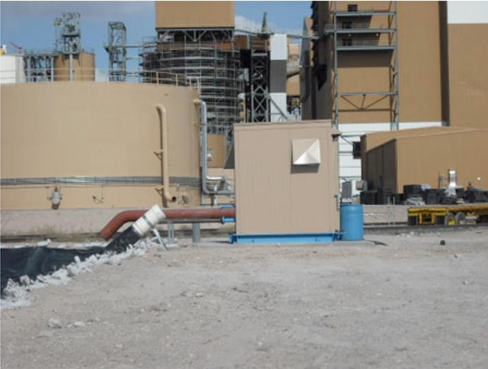
The effluent pond leak detection pumps lie on top of the secondary liner and are used only when, and if, the primary pond liner leaks. If a leak occurs, the level floats, and the pumps are activated. Submersible pumps centralized in a pipe with three Teflon® wheels were used for easy installation and servicing.
